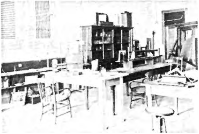
A typical installation modelled after Wundt's Leipzig facility; in this case the main psychological laboratory at Clark University, at the turn of the century. Clark University Archives.
